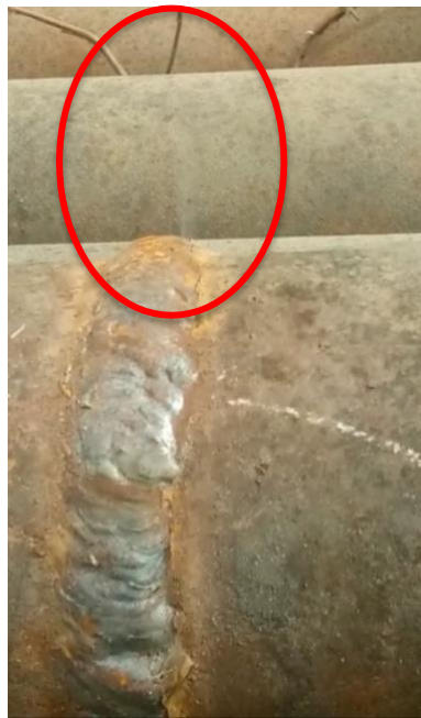
Photos: Gas leak continues; Gas leaking from welded section; Gas leaking from section tied with rag.
