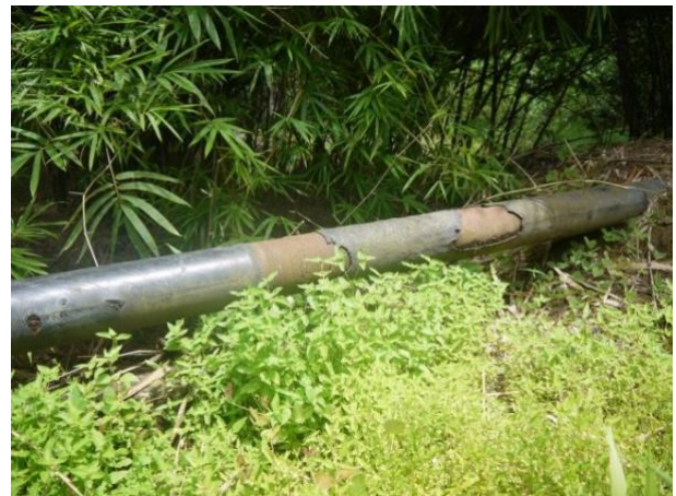
Photos: Gas pipelines running close to buildings; Overgrown pipelines with peeling surface layer (Source: SDN)
