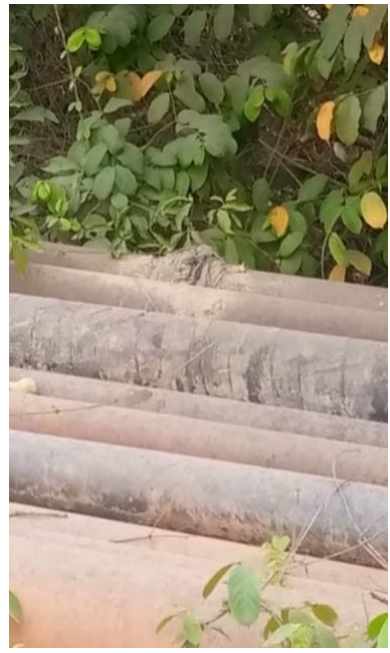
Photos: Gas leak continues; Gas leaking from welded section; Gas leaking from section tied with rag.
