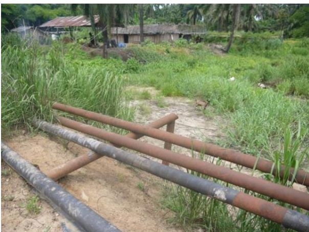
Photos: Gas pipelines running close to buildings; Overgrown pipelines with peeling surface layer (Source: SDN)
