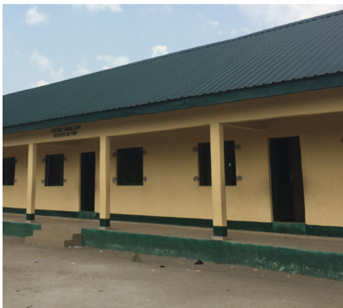
Nonwa's Community Secondary School, pictured here during repairs, was in dire need of renovation
